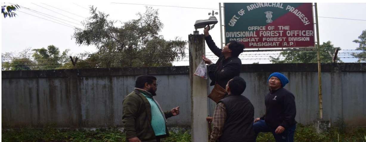
Pic 38 : AWS installed at DFO Office Pasighat
